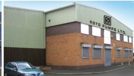
Manchester Office & Warehouse
